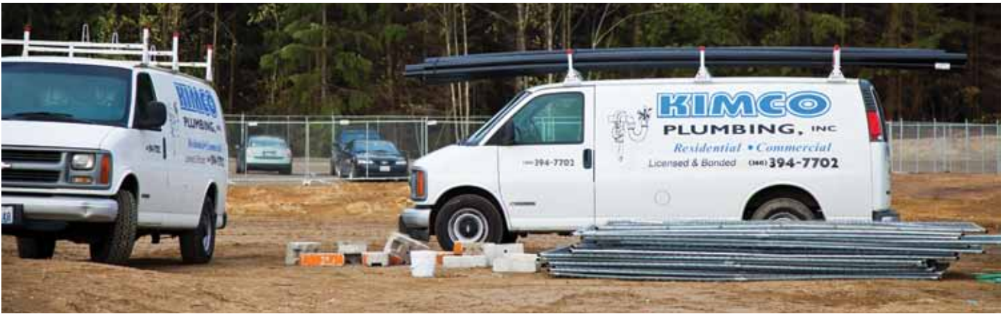
Poulsbo-based Kimco Plumbing at the Port Gamble S'Klallam Tribe's The Point Casino construction site.
