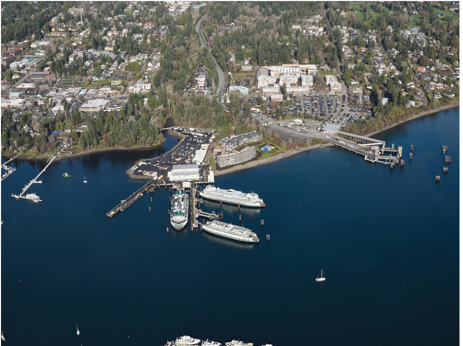
The Eagle Harbor Ferry Maintenance Facility on Bainbridge Island
